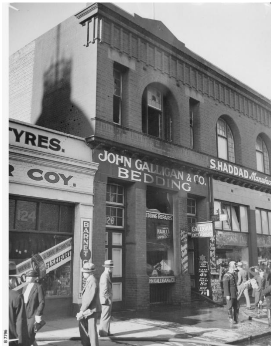
Grenfell Street [B 7796]. Grenfell Street, north side. The right side of the two storey building abuts Twin Street. The Grenfell Street frontage of the building is 17 yards. The photograph shows firemen cleaning up after a fire in the John Galligan Bedding Store. Windows are blackened and broken and a hose and water is coming out of the doorway. 1938. Henry Krischock, Part of Acre 102 Collection
