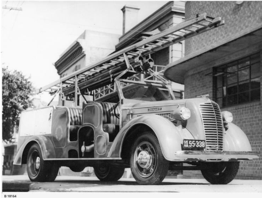
State Library of South Australia - Fire Engine [B 10164], The new Fire Engine for the South Australian Fire Brigade Board equipped with a 40 ft. extension ladder and a 2,000 ft. hose. Seating capacity: 6. Pump capacity: 400 gallons a minute. This model is a Diamond and the South Australian registration number is 155-338. 1938. Photographer, News and Mail, Part of General Collection.
