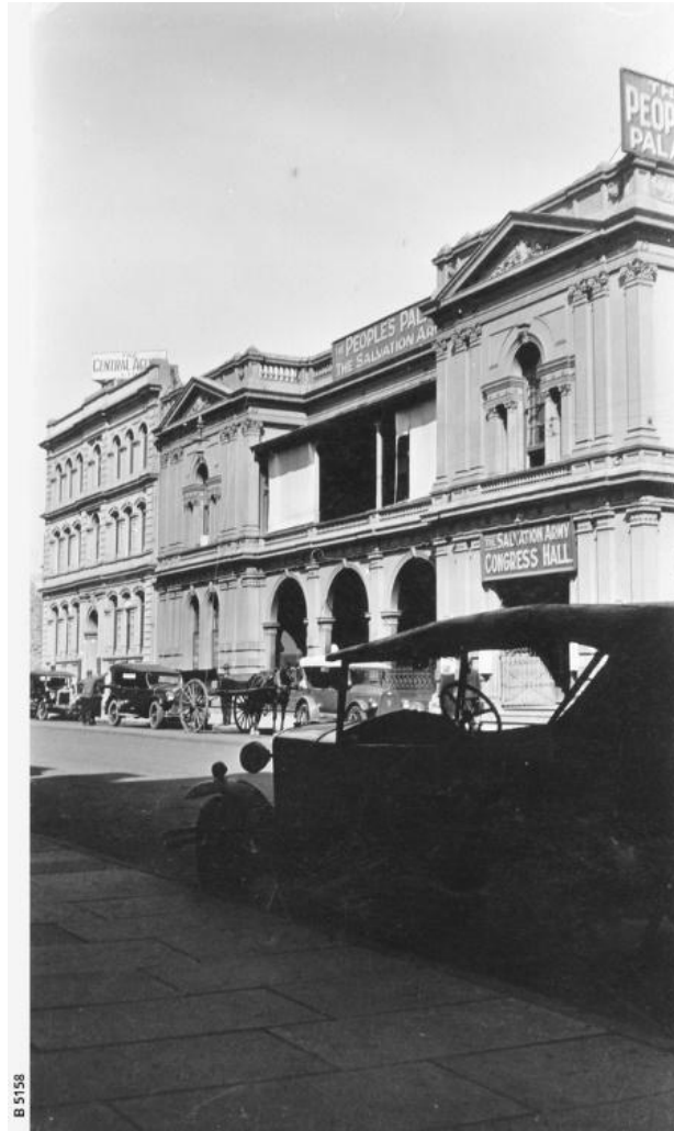
State Library of South Australia - Pirie Street, People's Palace for the Salvation Army [B 5158], Pirie Street, south side, March 13th 1929. For alterations and additions made to the People's Palace in 1938 see B 8189. Site of the People's Palace: near side is 12 yards west of Chesser Street. Frontage 33 1/2 yards. The roofed balcony was added in 1911 according to HT Griggs, Architect. Salvation Army Congress Hall. 1929. Photographer, State Library of South Australia.
